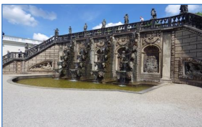
The water cascade at Herrenhausen
